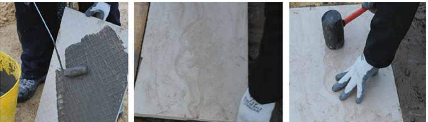
**We recommend that Vitripiazza is only installed using Pavetuf Priming Slurry and jointed with either our Jointing Mortar or Jointing Compound. If these products are not used for Vitripiazza installation purposes, the integrity of the paved system is outside our recommend guide and will forfeit any technical support.**
